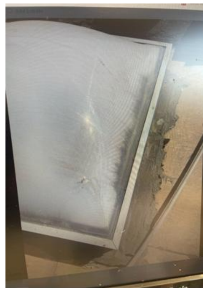
Damaged Skylight
